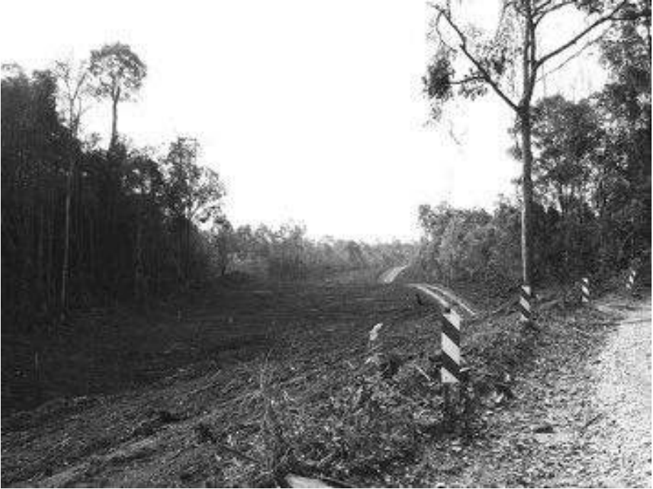
Figure 4.5 Excessive road clearance
