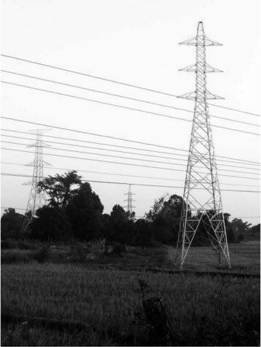
Figure 4.1 Nam Theun 2 Transmission tower
